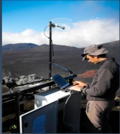
Installation of a GPS station on Piton de la Fournaise (UnderVolc - IPGP)
